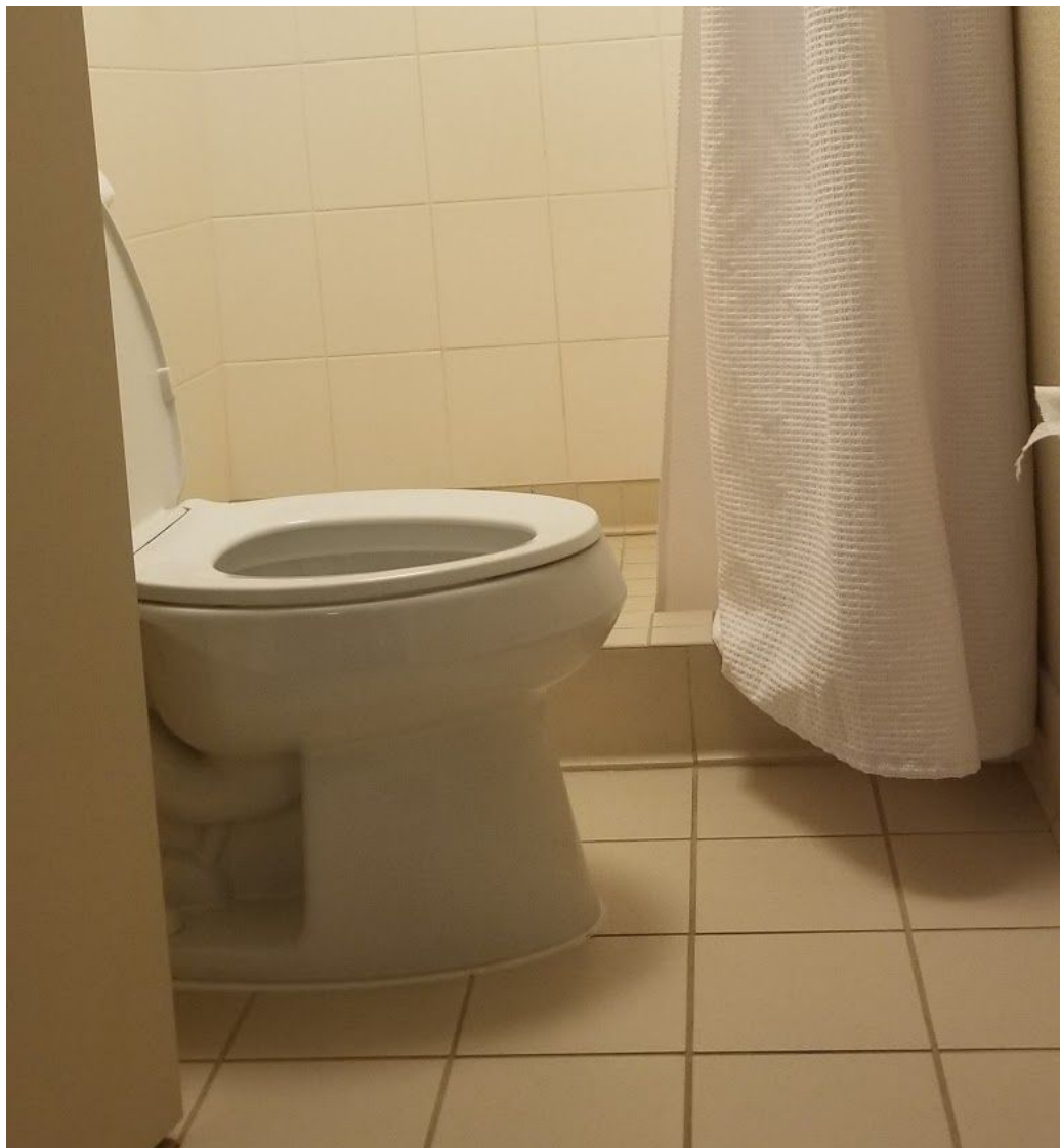
Image 15: Springhill Suites by Marriott bathrooms with only a shower have a lower shower lip, making it easier to get in and out of the shower, if a roll in shower is not required.
