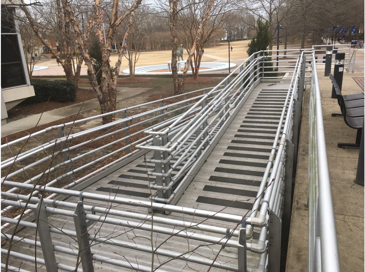
Image 1: Webb Center entrance ramps have metal railing and traction tape. Ramps zig zag back and forth.
