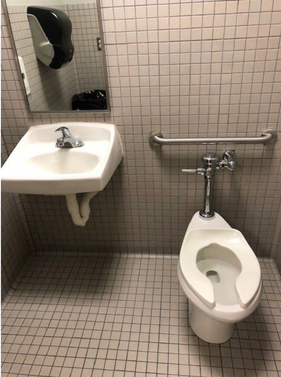
Image 7: Private, gender neutral bathrooms. Bathroom includes hand railing, toilet paper, and paper towels that are all at accessible levels. These bathrooms are much more accessible and have more room than the multi-stall Men and Women restrooms.
