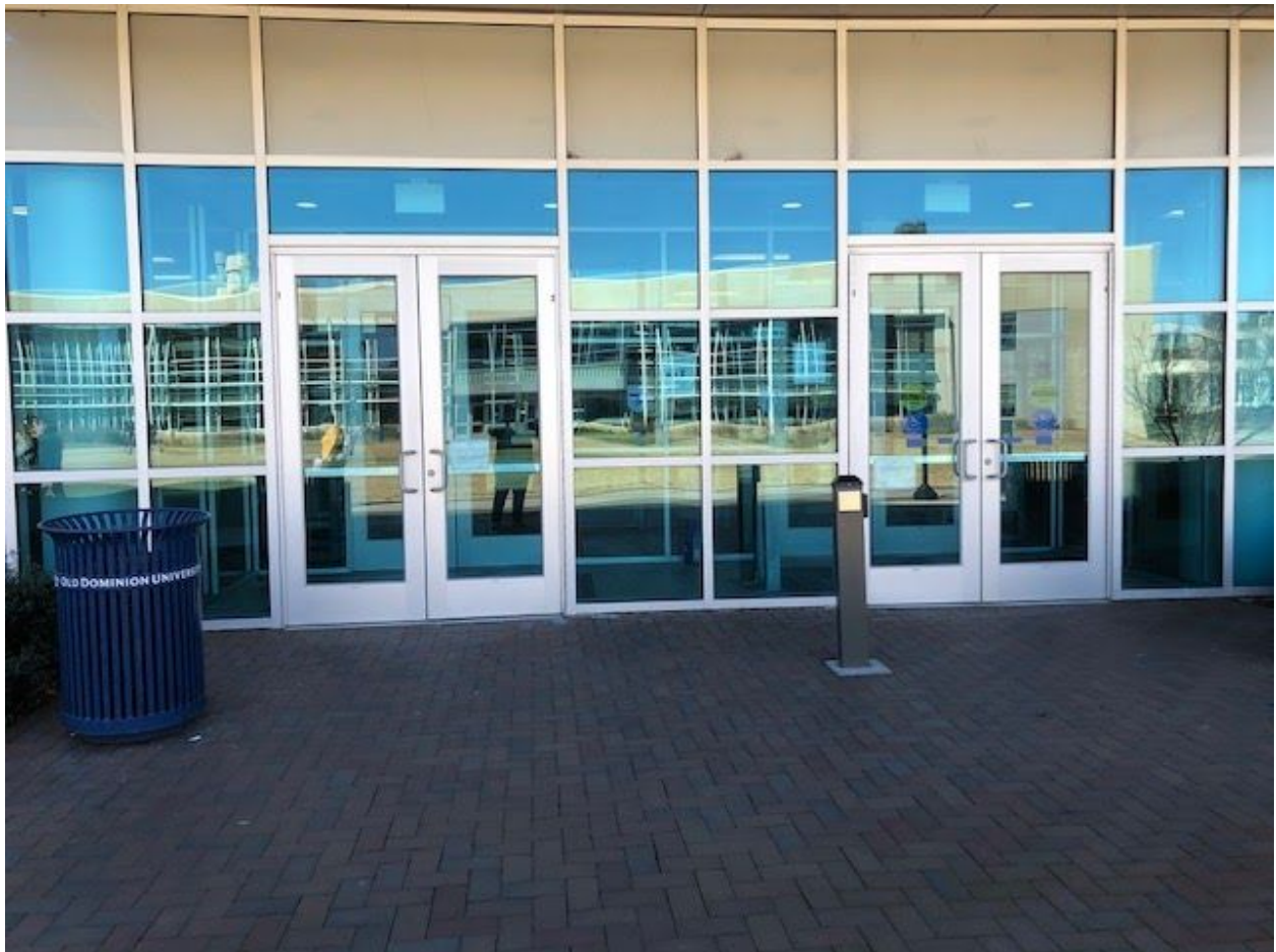
Image 4: Front entrance to the library. The doors on the right are controlled by the automatic door opener located left of the right side doors. There are two sets of doors in order to enter the library. Ramps are located to the left and right sides past the second set of doors.
