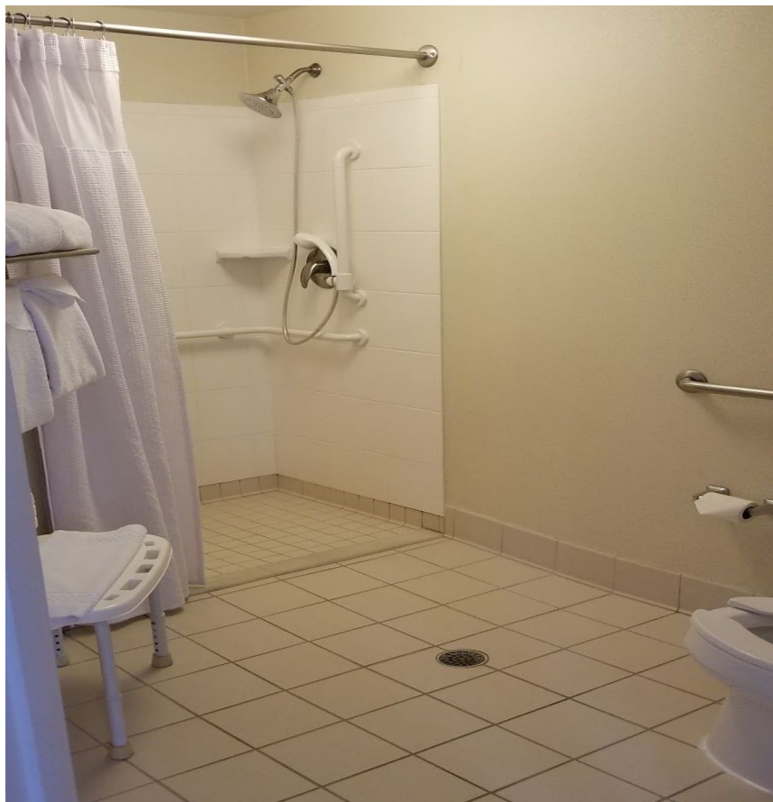
Image 14: Accessible bathrooms in the Springhill Suites by Marriott include a roll in shower with hand rails, a hand-held shower head, and a shower chair. There is also hand railing near the toilet.
